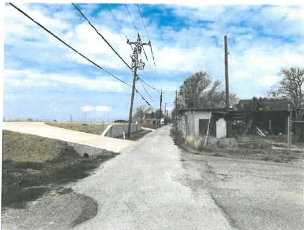
VIEW FACING WEST ALONG NORTH FRONT STREET
