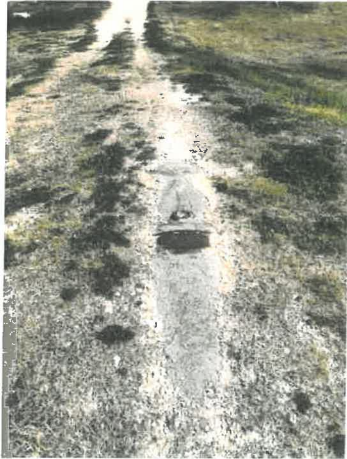
VIEW OF STORM DRAIN CULVERTS EXTENDING FROM RIVER TOWARD FRONT STREET
