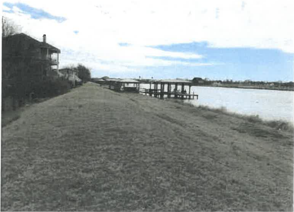
VIEW OF OLD BRAZOS RIVER LEVEE ACROSS SITE
