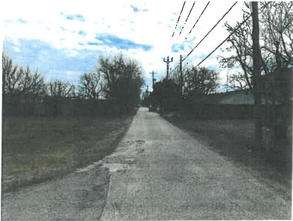
VIEW FACING EAST ALONG NORTH FRONT STREET
