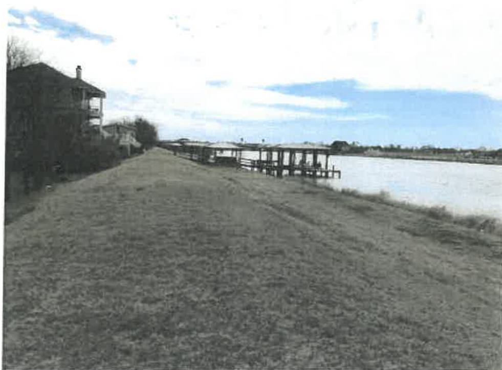
VIEW OF FOLD BRAZOS RIVER LEVEE ACROSS SITE
