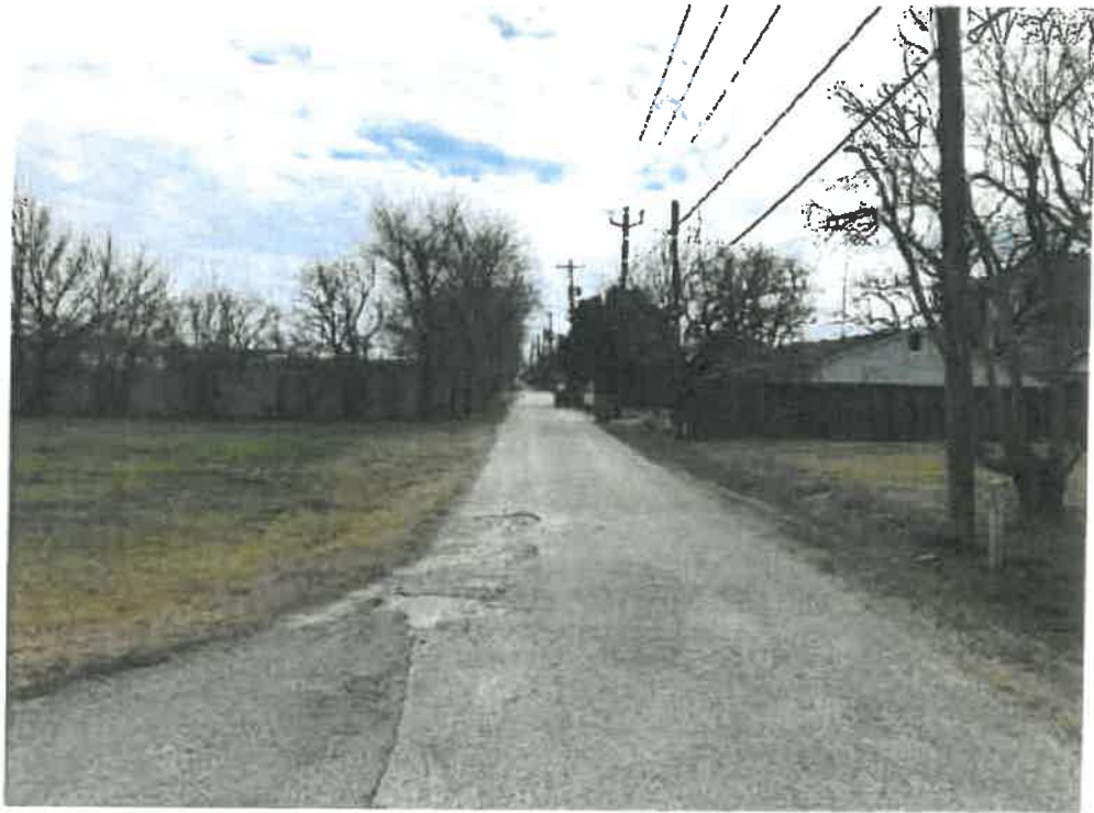
VIEW FACING EAST ALONG NORTH FRONT STREET
